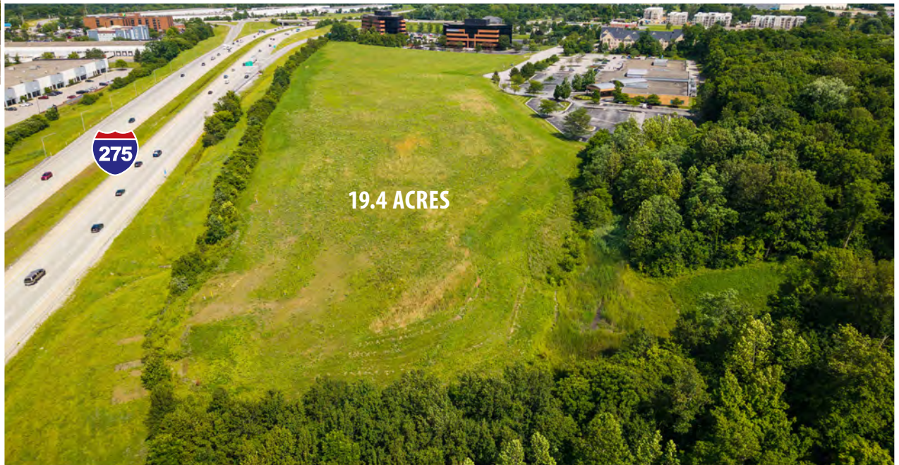
Aerials 7.2.2025 Cleared & Graded
